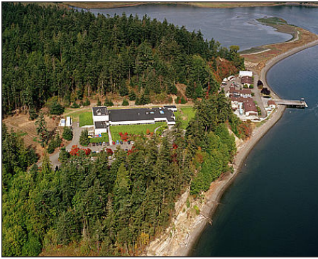
The PNNL Marine Sciences Laboratory in Sequim is using two of its backup generators for the distributed generation portion of the program.
